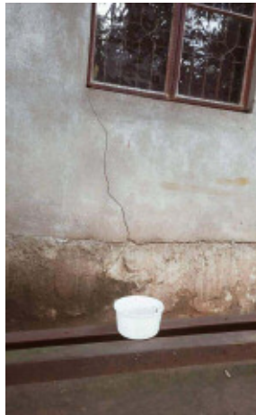
Damage caused by water seepage under the monastery
