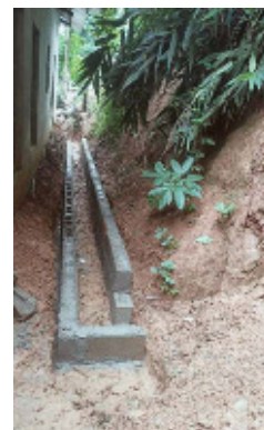
Received June 13, completed construction of a drain beside the monastery
