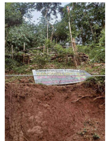
A landslide at the site for the stupa above the monastery
