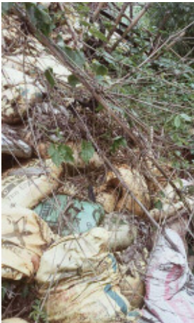
Collapse of some of the reconstruction work
