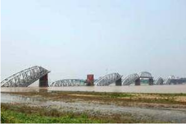
The collapsed Ava Bridge in Mandalay [EPA]
