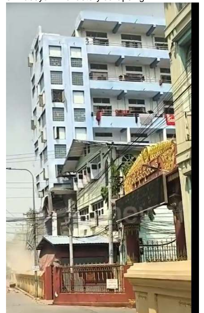
Click the image below to watch a graphic video of Masoyein Monastery collapsing
