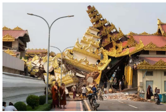
The collapsed Maha Myat Muni Pagoda in Mandalay / EPA
